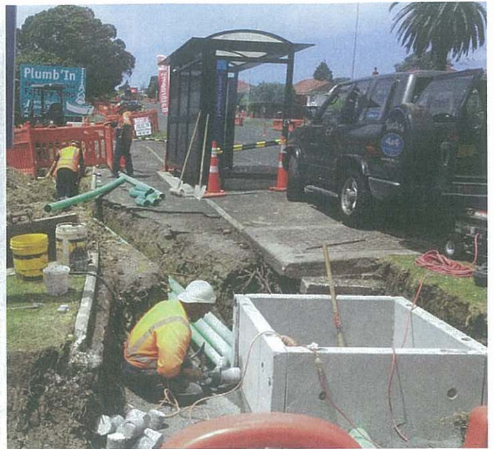
The fitting of an underground service chamber on Wolverton Street
