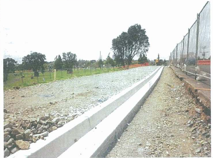
New kerb and channel near Olympic Park
