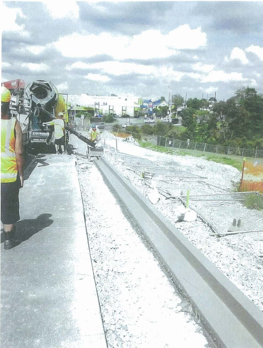
The laying of new kerb and channel along Wolverton Street
