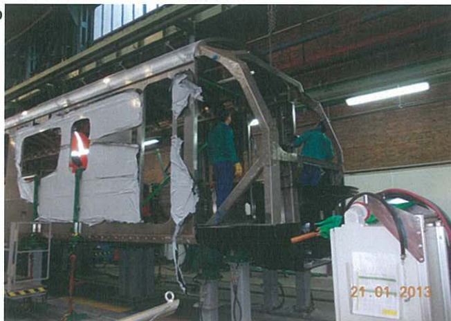
Fig 3: Cab Framing fitted to the first vehicle
