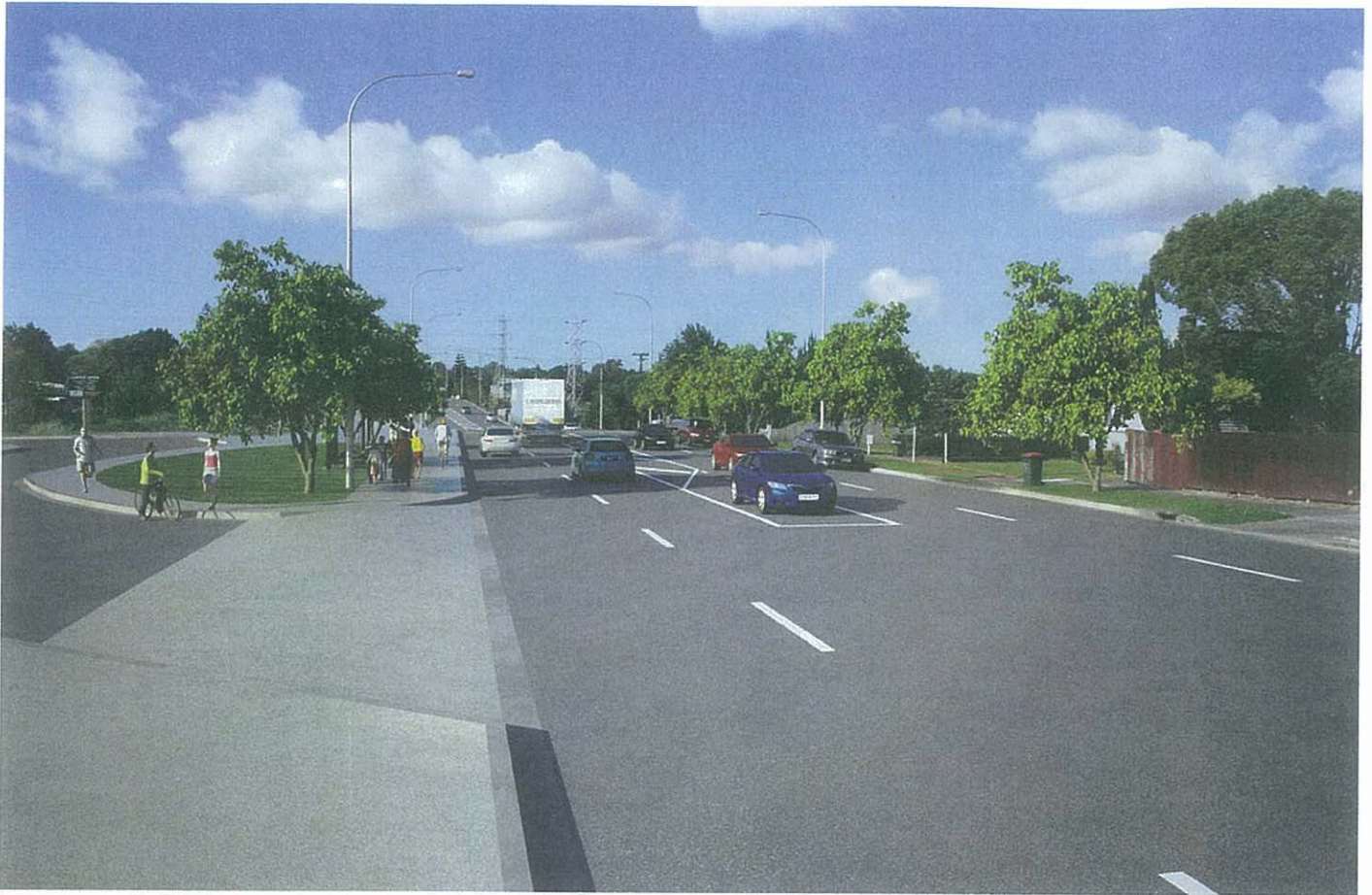
An indicative view of a completed section of Wolverson Street by Olympic Park
